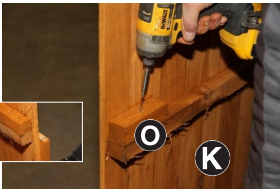
28. Fix Part O to Part K internal baton flush with Part K baton as shown in image using 2no 60mm screws. Repeat on opposite side door.
