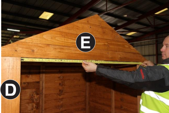
11. Before fixing Part E across Part D on opposite side ensure there is a gap of 1360mm between both front panels top and bottom to fit door.
