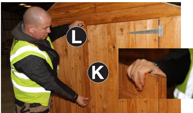
30. Fit Part L to right hand side of Part K flush with top and centralise on joint between both doors using 3no 25mm screws top, bottom and centre.
