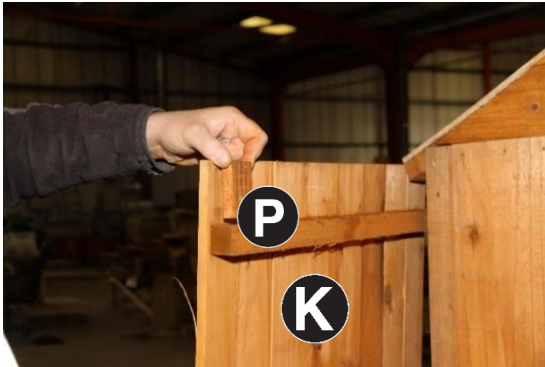
26. Attach Part P in line with baton as per image using 1no 25mm screw
