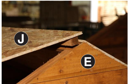
22. Place roof panel Part J onto both Part E gable ends ensuring overlapped side hooks onto Gable E. Repeat on both sides of shed.
