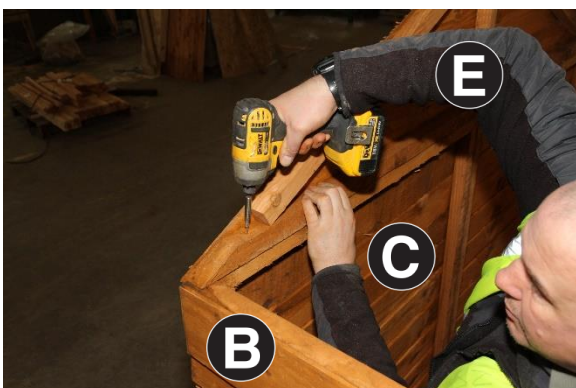
15. Fix Part E to Part C using 1no 60mm Screw. Repeat both sides.
