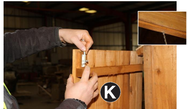
27. Attach slide bolt us 4no 25mm screws as above image.
