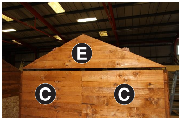
14. Place Part E across both Parts C back panels edge to edge.
