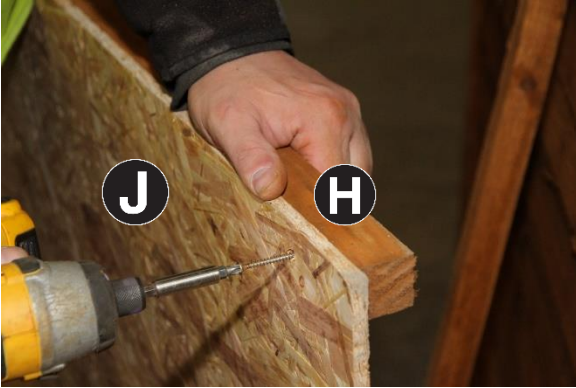
19. Attach Part H to Part J to the longest length flush with edge leaving an evenly spaced gap either end. Fix together using 4no 40mm screws. Repeat on second panel.
