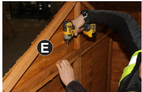
16. Fix Part E to Part C using 1no 60mm Screw as shown. Repeat both sides.
