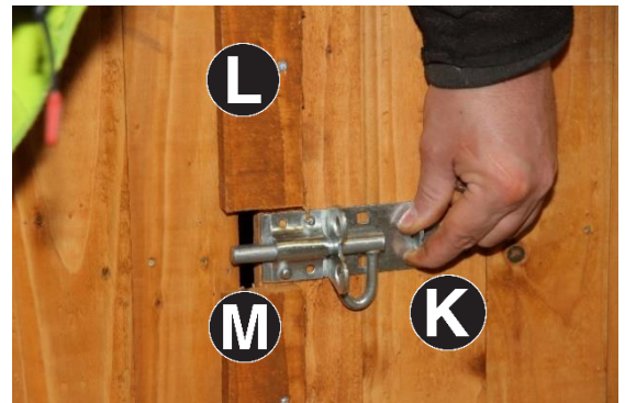
31. Attach Pad Bolt to right hand side of part K in-between Part L and Part M as per image using 4no 25mm screws
