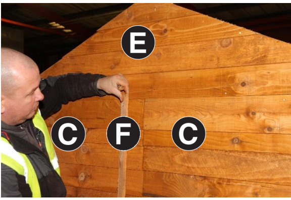
17. Attach Part F cover strip to Centre of both Part C's starting at bottom of Part E using 3no 40mm screws top, bottom and centre.
