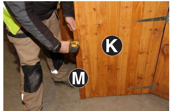
29. Fit Part M to right hand side of Part K flush with bottom and centralise on joint between both doors using 3no 25mm screws top, bottom and centre.
