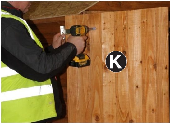
24. Align hinges with batons and fix to Part K using 4no 25mm screws per hinge. Repeat on next door (3 hinges per door).
