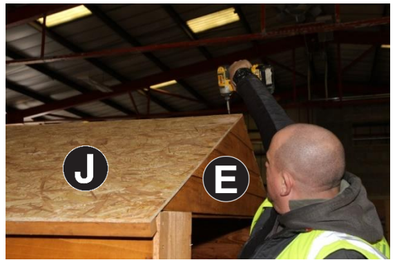
23. Line up Part J roof panel with Part E gable, using 3no 40mm screws screw into Part E repeat on all four sides.
