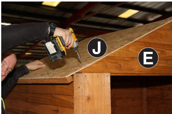
23. Line up Part J roof panel with Part E gable, using 3no 40mm screws screw into Part E repeat on all four sides.
