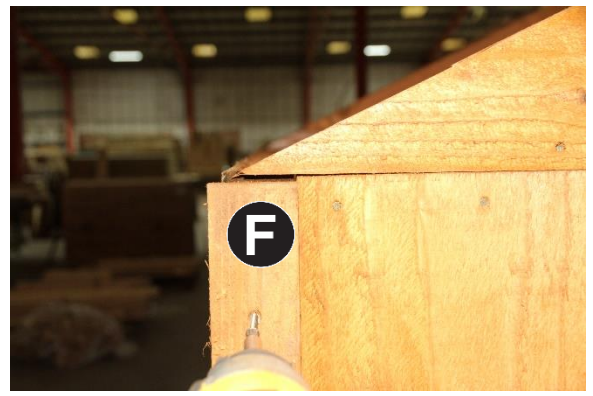
18. Fix Part F to all four corners of the shed leaving 10mm space from the top using 3no 40mm per corner top, bottom and centre.
