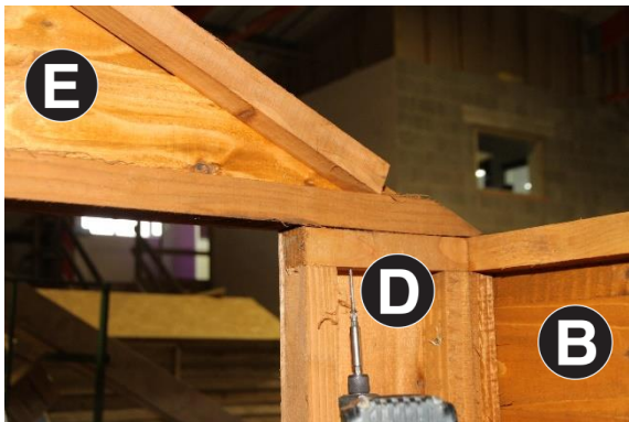
13. Once Part E is fitted screw part D to Part E internally as per image. Repeat on opposite side
