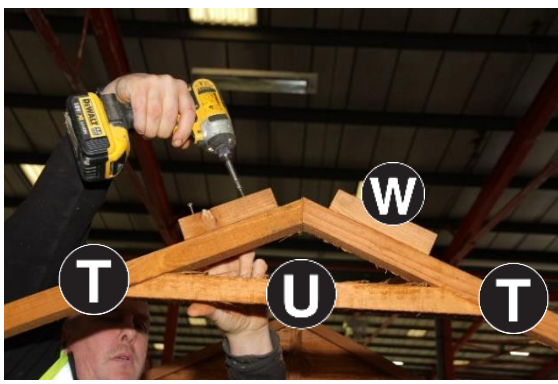
25. Attach Part W to Part T using 2no 60mm screws spaced evenly 40mm from apex as shown on image. Repeat on both sides.
