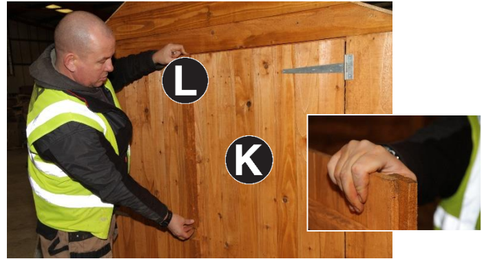
38. Fit Part L to right hand side of Part K flush with top and centralise on joint between both doors using 3no 25mm screws top, bottom and centre.
