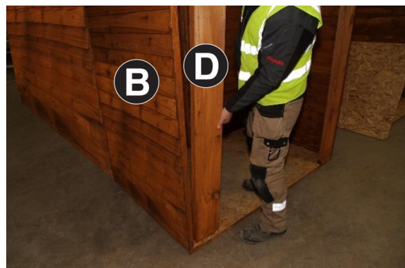
8. Attach Panel D to Panel B using 3no 60mm Screws. 100mm from top, 100mm from bottom and one in the centre. Repeat on opposite side.
