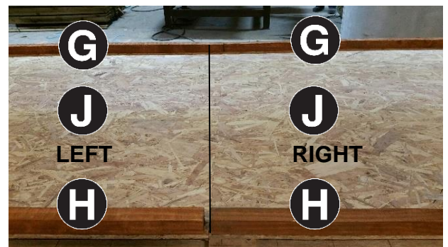
28. Attach Part G to Part J leaving the sheet overhanging 14mm. On two panels, Part G should be flush on right hand side of Part J. The two other panels should be flush on left hand side of Panel J. See images below for finished roof panels.
