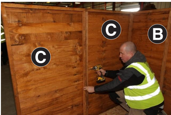
5. Fix second piece of Part C to first piece using 3no 60mm Screws. 100mm from top, 100mm from bottom and one in the centre.
