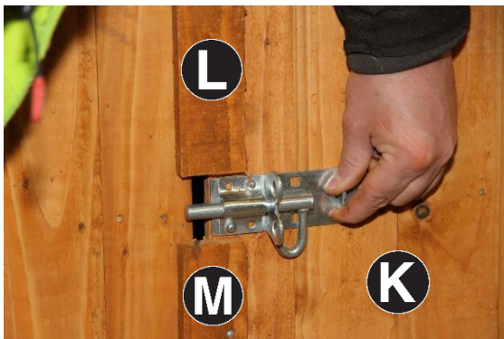
39. Attach Pad Bolt to right hand side of part K in-between Part L and Part M as per image using 4no 25mm screws
