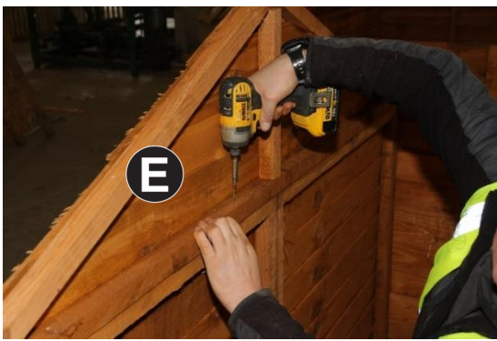
17. Fix Part E to Part C using 1no 60mm Screw as shown. Repeat both sides.
