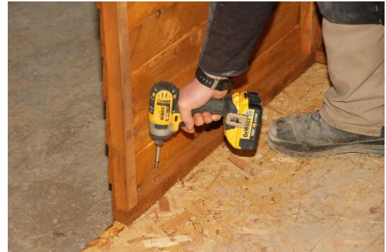
20. Fix all panels to floor using 2no 60mm screws per panel.
