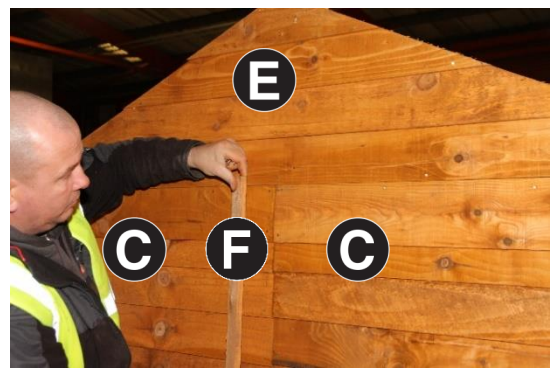
18. Attach Part F cover strip to Centre of both Part C's starting at bottom of Part E using 3no 40mm screws top, bottom and centre.
