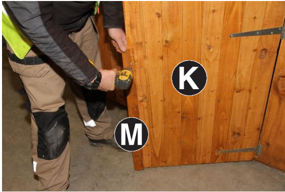
37. Fit Part M to right hand side of Part K flush with bottom and centralise on joint between both doors using 3no 25mm screws top, bottom and centre.
