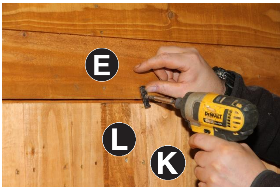
41. Attach Turn Button Latch to Part E using 1no 40mm screw as per image.
