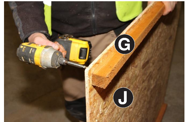
28. Attach Part G to Part J leaving the sheet overhanging 14mm. On two panels, Part G should be flush on right hand side of Part J. The two other panels should be flush on left hand side of Panel J. See images below for finished roof panels.
