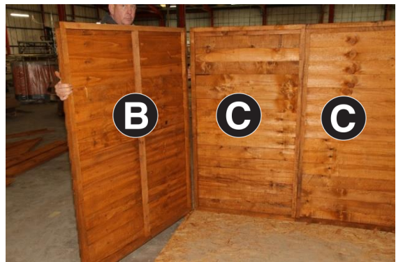
6. Fix second piece of Part B to second piece of Part C using 3no 60mm Screws. 100mm from top, 100mm from bottom and one in the centre.
