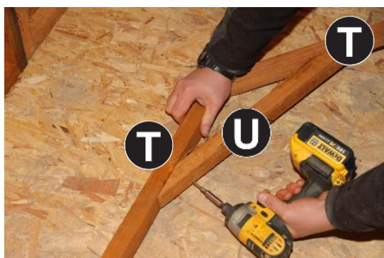
23. Fix Part U to Parts T using 1no 60mm screw. Repeat on other side.
