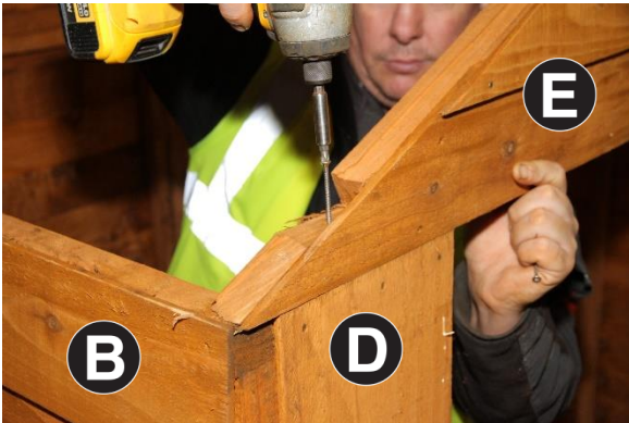
11. Place Part E across Part D and align with opposite corner of Part B. Screw together using 1no 60mm screw.
