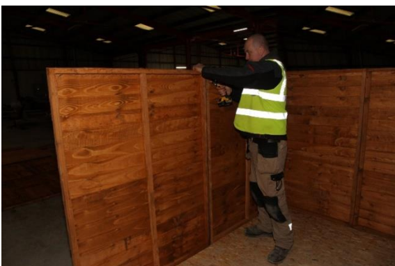
7. Fix second piece of Part B to other Part B using 3no 60mm screws as per image.
