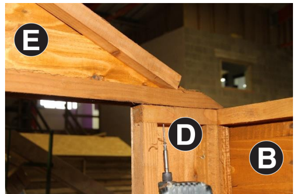
14. Once Part E is fitted screw part D to Part E internally as per image. Repeat on opposite side
