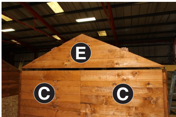
15. Place Part E across both Parts C back panels edge to edge.
