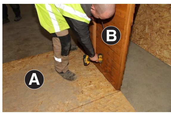
2. Place Part A on a flat surface and attach Part B using 2no 60mm Screws.
