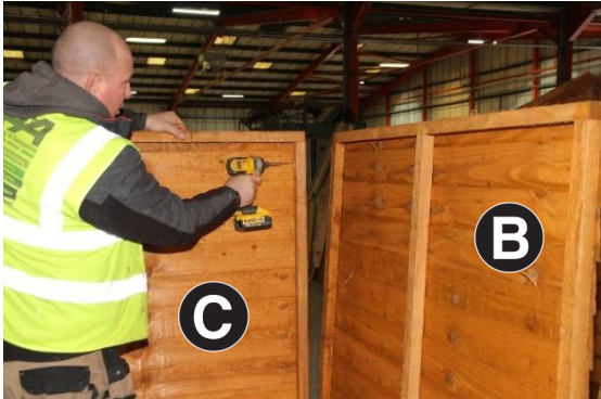
3. Fix first piece of Part C to Part B using 3no 60mm Screws. 100mm from top, 100mm from bottom and one in the centre.
