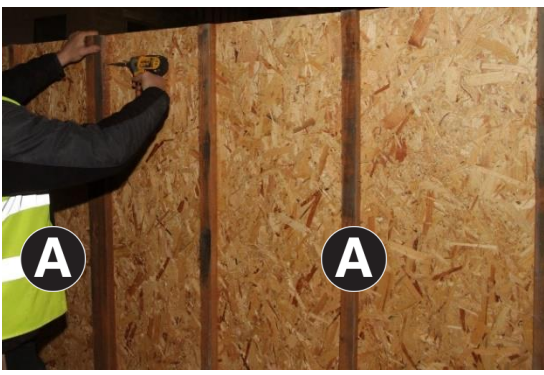
1. Place both Part A's together as per image using 4no 60mm Screws, top bottom and spaced evenly.
