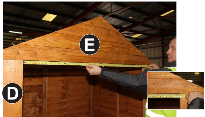
12. Before fixing Part E across Part D on opposite side ensure there is a gap of 1360mm between both front panels top and bottom to fit door.
