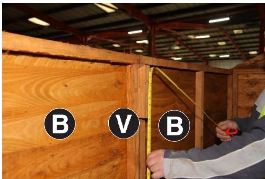
21. Fix Part V with lower angle facing Part B measuring 1353mm from floor using 2no 60mm screws fix right hand side bottom then left hand side top to ensure good fix between both panels as per image. Repeat on both sides.
